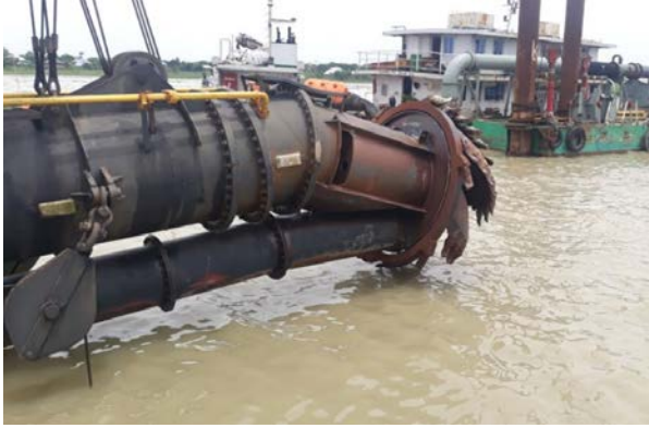
Operation of Cutter Suction Dredger near Padma Bridge, Shimulia
