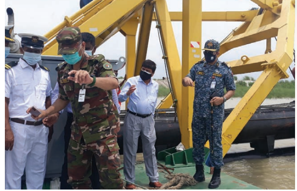
Inspection of Cutter Suction Dredger near adma Bridge, Shimulia
