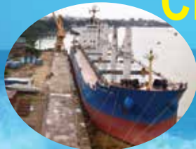
Jetty Service and Berthing Facility
